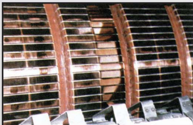
Figure 11 Stripping – Less film on the fourth brush path is a destructive condition. The slot bar pattern is acceptable since the bars are not etched.
